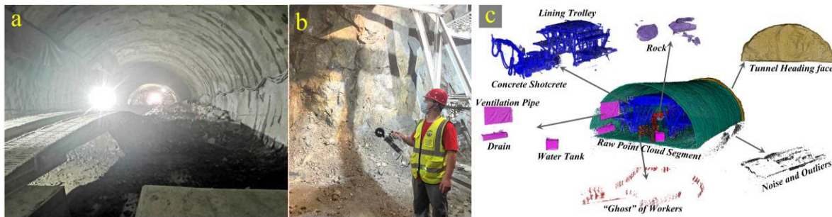
Figure 1. (a) The tunnel construction site; (b) Tunnel 3D point cloud data is being collected using HLS on the site ; (c) Complex point cloud data of tunnel construction site (Cui, 2023).
